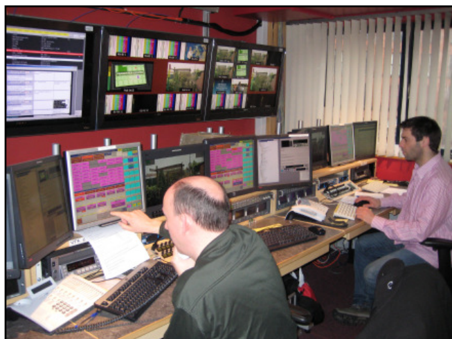
BBC Belfast facility
